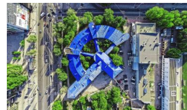
The kitchen factory building
